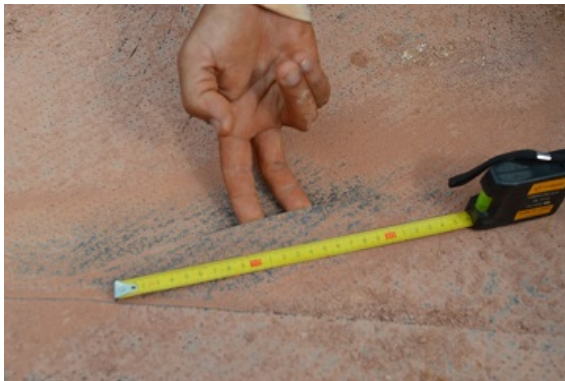
Figure 5. Cut damage.
