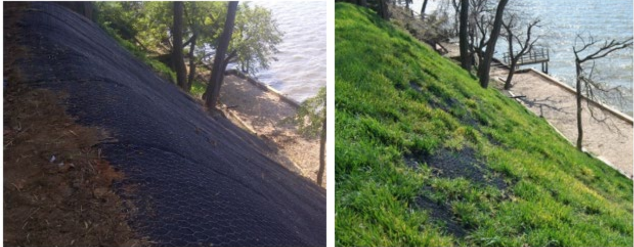
Figure 2. Geomat with DTWM reinforcement on a steep soil slope before and after the establishment of vegetation.
