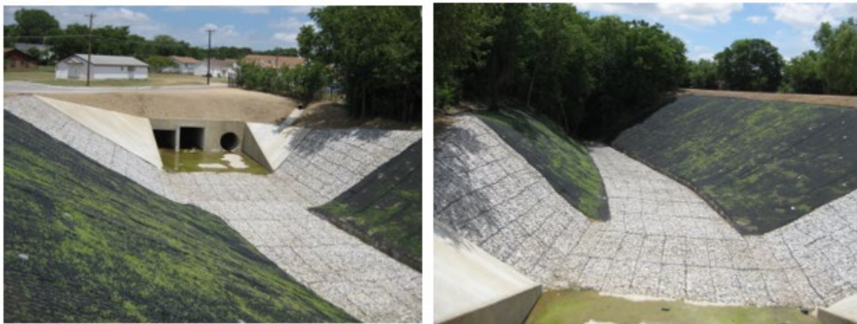
Figure 5. Geomat with DTWM reinforcement hydraulic application.
