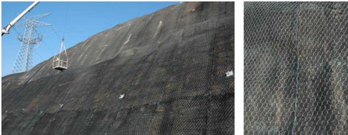
Figure 3. Connection of geomat with DTWM adjacent rolls without overlapping detail.
