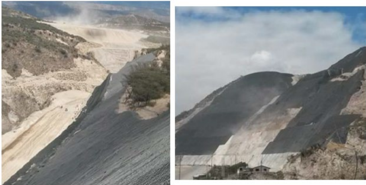
Figure 6. Installation of a geomat with DTWM reinforcement on a rocky slope.
