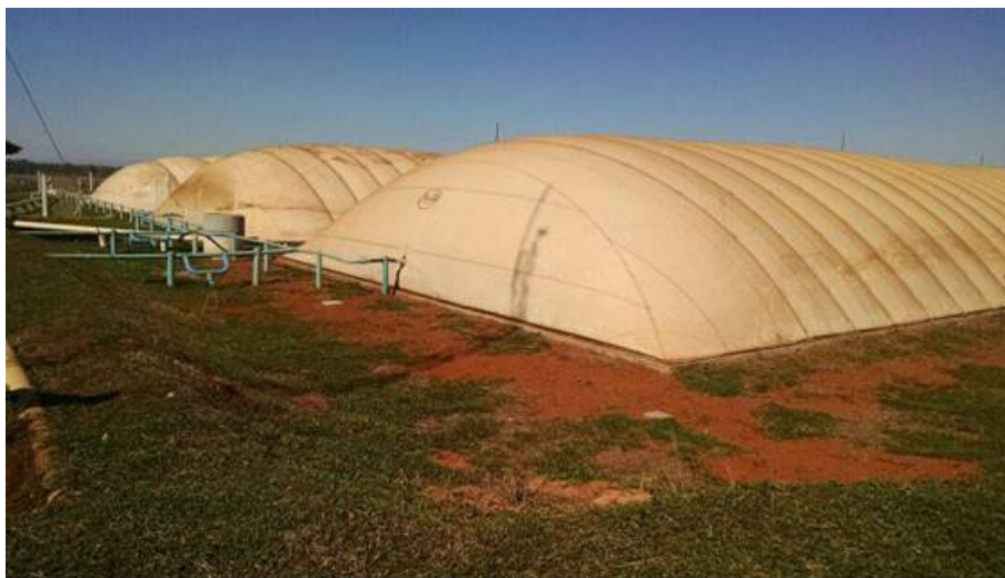
Figure 3. Gas outlet pipe.
