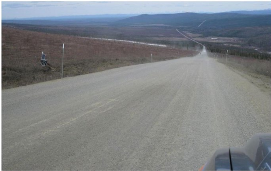
Figure 7. Post Active Drainage Geosynthetic Installed Section.
