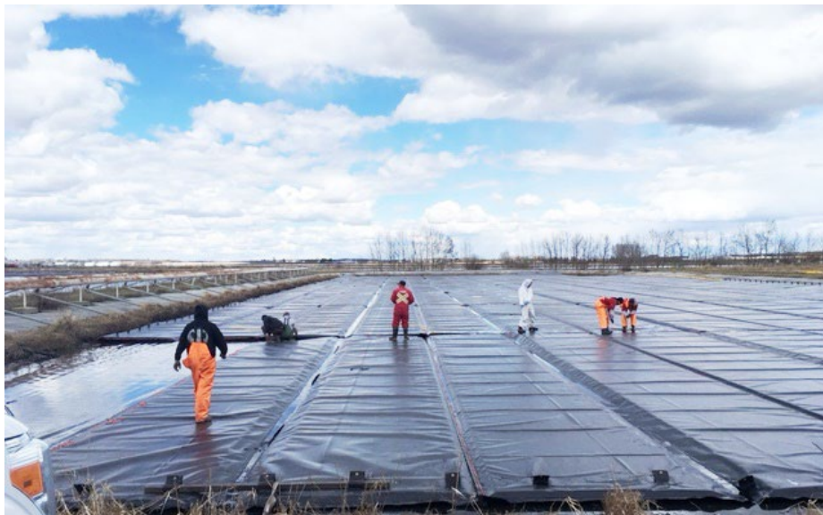
Figure 9. Geosynthetic Technicians walking on the cover during panel deployment
