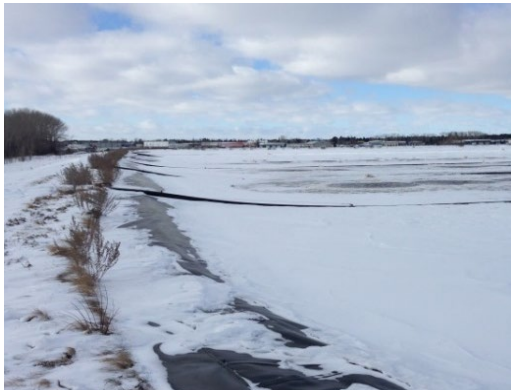
Figure 5. Snow and Ice build-up
