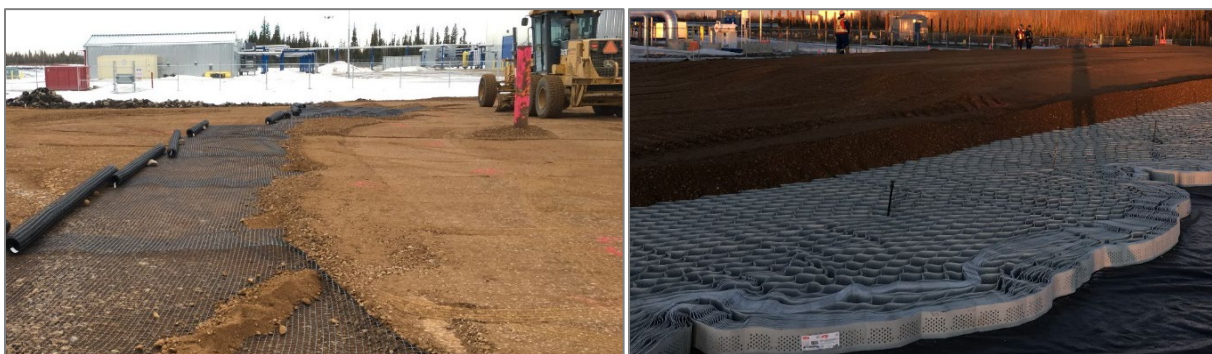
Figure 3: a) Partially filled geogrid Layer and b) Partially filled top NPA geocell layer
